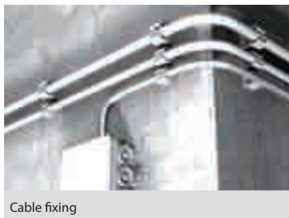
Fixing plastic insulating conduits
